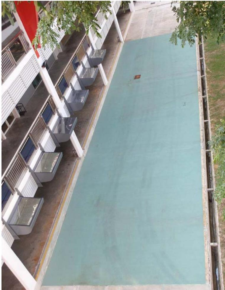
**The application of cool pavement coating (blue color pavement), and mirror ducts at the side of the building for the rooms natural lighting**
