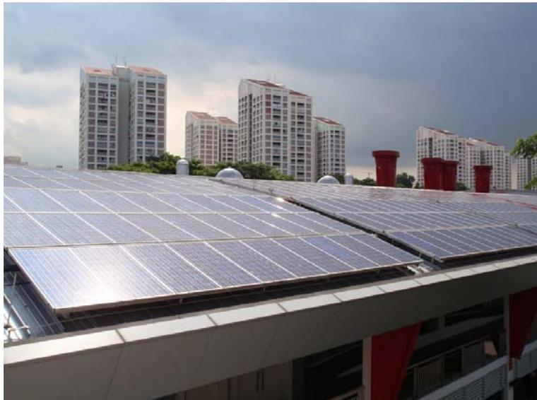
**Solar chimneys and full coverage of solar panels at the rooftop of ZEB**
